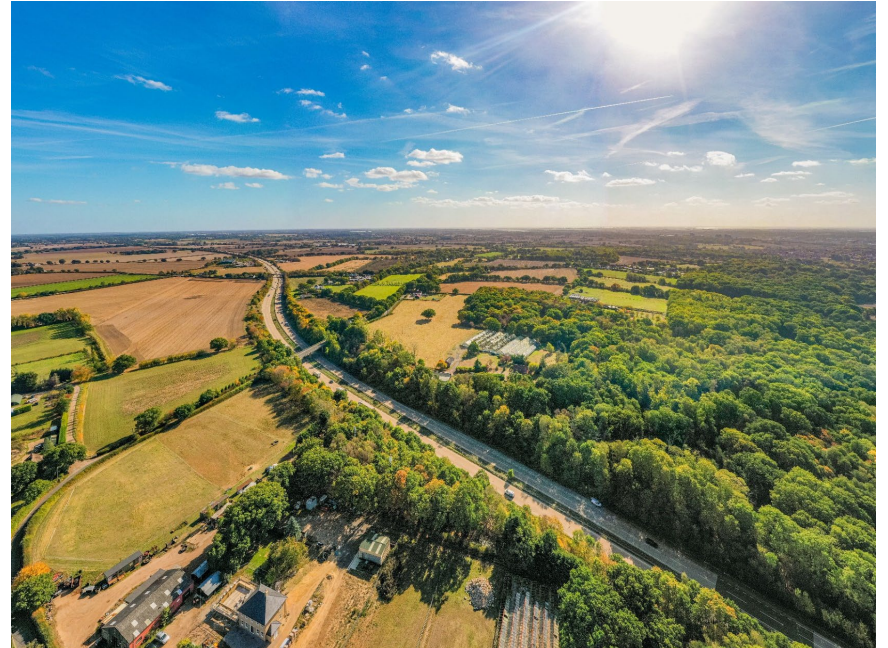
Above: Drone photography of TCBGC site area, with A120 heading east in the centre of the image.
